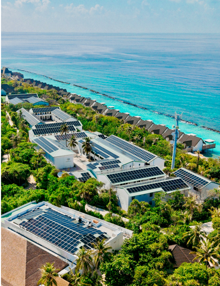
Solar Panel Installation at Meyyafushi Maldives
